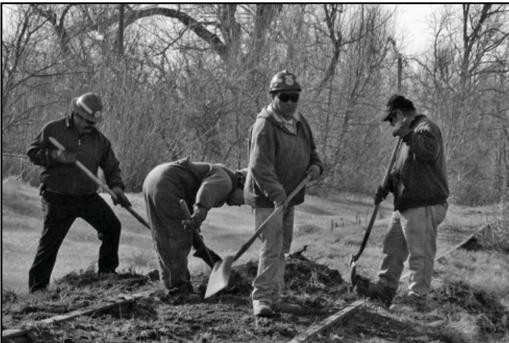
Some of Bob Hussey Construction crew removing overgrowth prior to tamping
